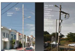
The next day after building a "Small Cell" the carrier can use a Federal law to add more antennas and cabinets on the ground or pole. As well as additional height (10-20 feet) and width (6+ feet) and more antennas
