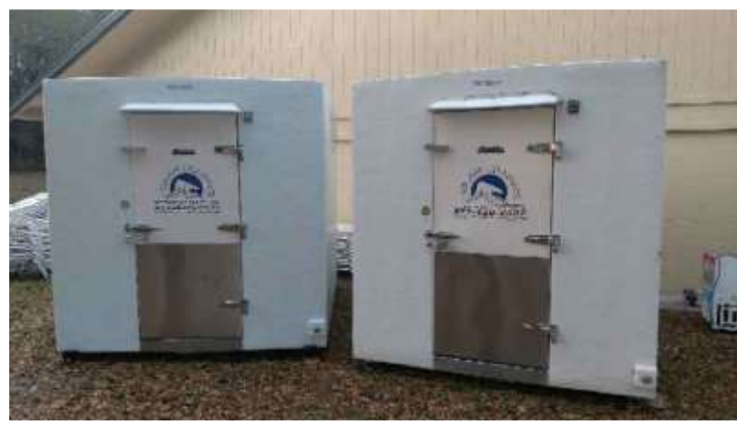
Walk-In Cooler & Freezer
